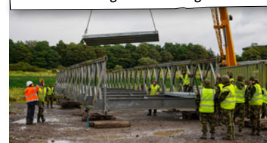
Engr: Students on a Combat Engineers course learning to build bridges
