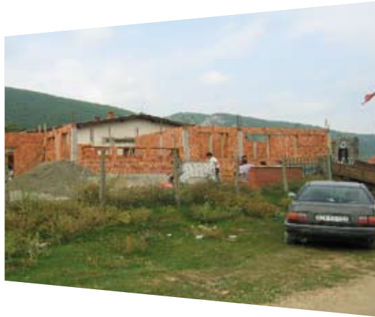
Renovations to local school in Banjica in progress.
