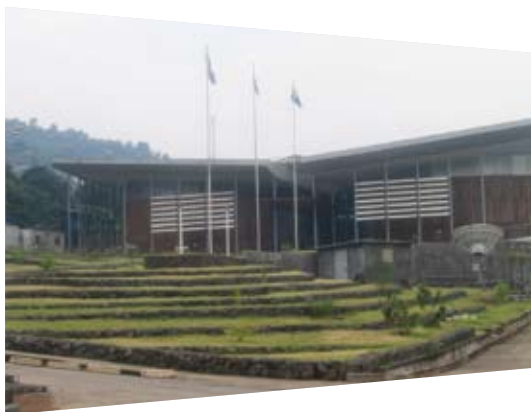
Special Court for Sierra Leone building in Freetown.
